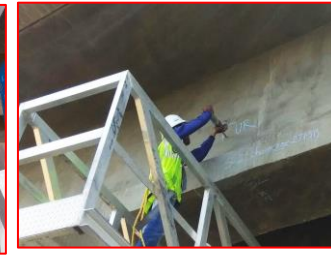
Use of Mobile Bridge Inspection Unit (MBIU)
