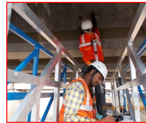
Use of Mobile Bridge Inspection Unit (MBIU)
